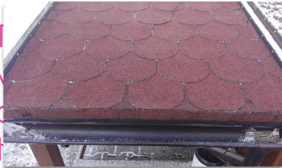
Roof with asphalt shingle
